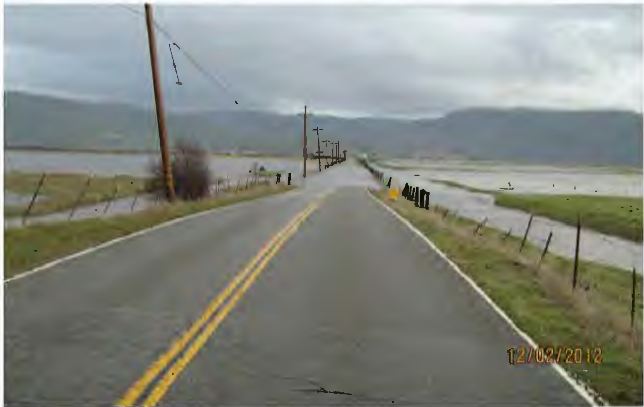
Figure 4-119 Indian Valley Localized Flooding – Ponding area of Stampfli Lane has Poor Drainage and Floods Annually
