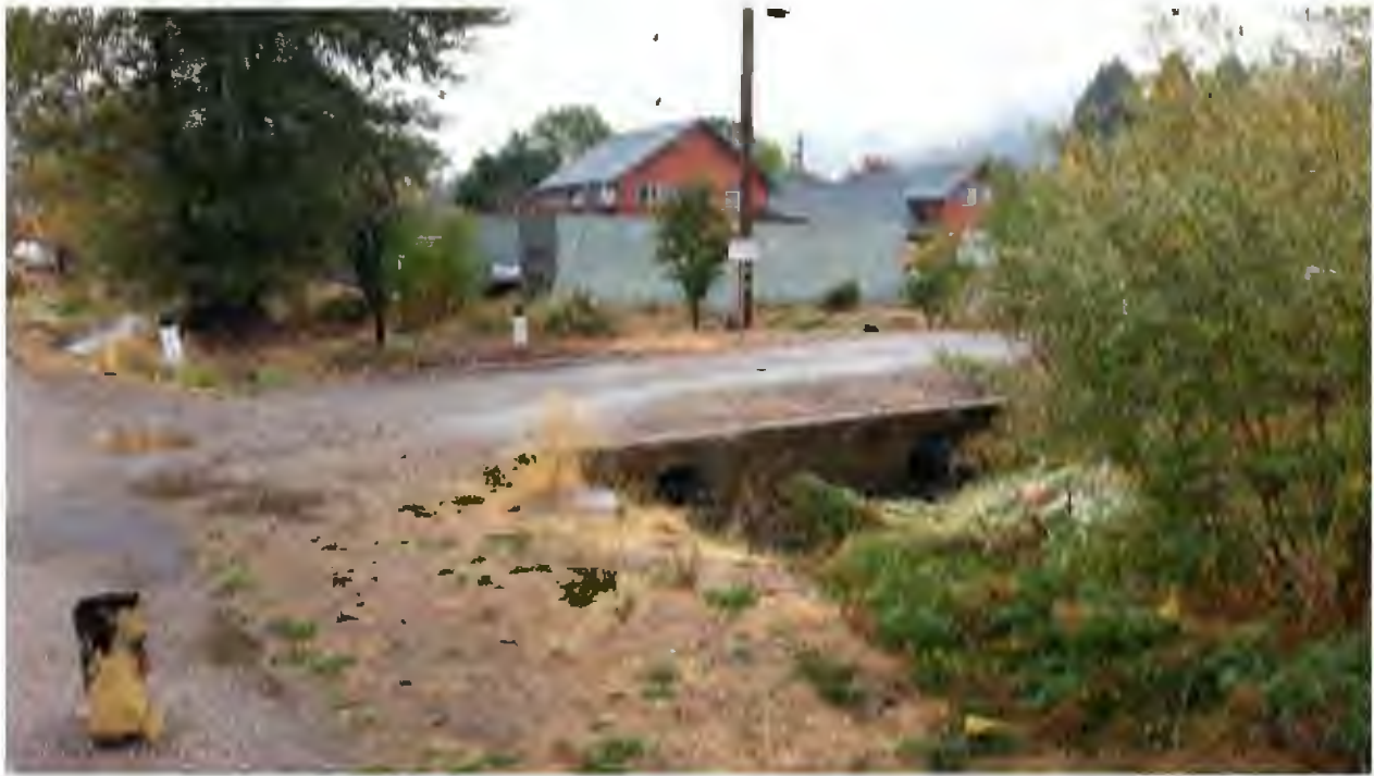
Figure 4-128 American Valley Localized Flooding – Water Overtops Drainage at Culverts Where Forced to take 90-degree Right Turn.
