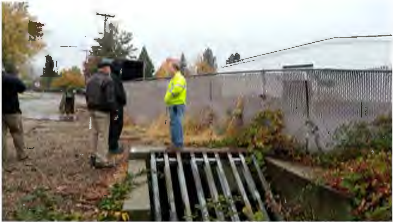
Figure 4-123 American Valley Localized Flooding – Storm Grate behind Les Schwab Becomes Clogged with Debris Causing Flooding
