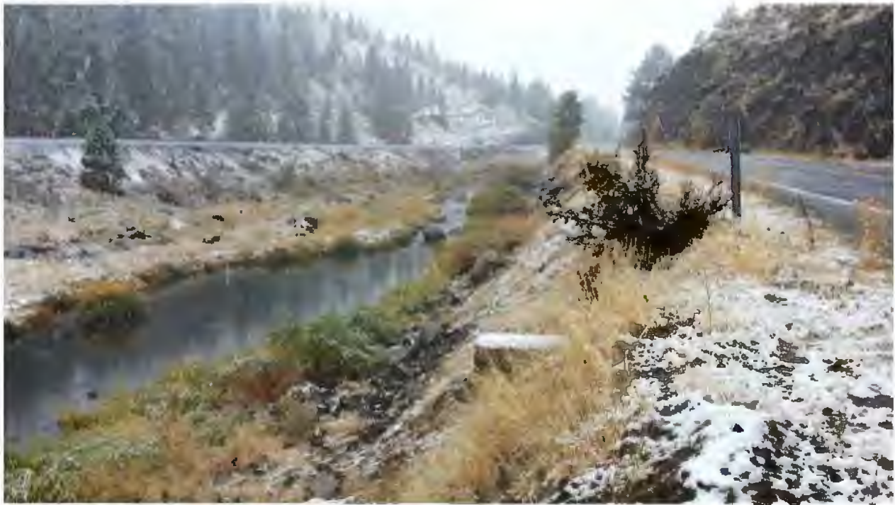
Figure 4-116 Rocky Point Road – Shoulder Erosion from Localized Flooding
