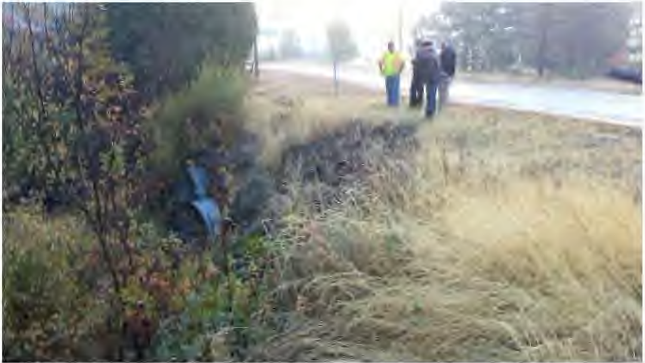
Figure 4-118 Indian Valley Localized Flooding – North Valley Road crossing Williams Creek where Culverts often Clog with Debris
