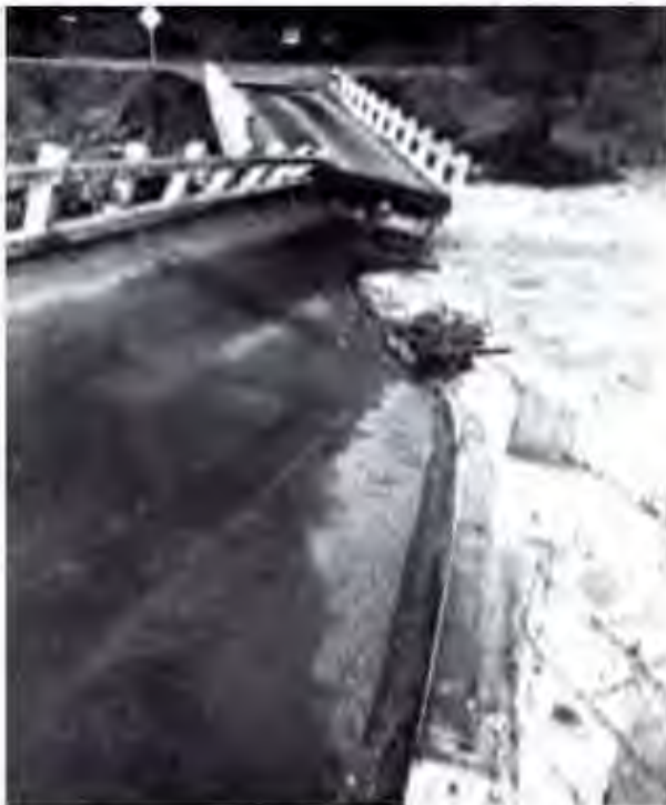
Figure 4-93 Bridges Destroyed by Flooding – Indian Creek Bridge (left) and Mohawk Valley Bridge (right)
